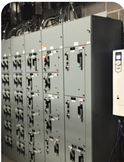
Installation & Commissioning of ABB VFDs – Aramco, Riyadh
