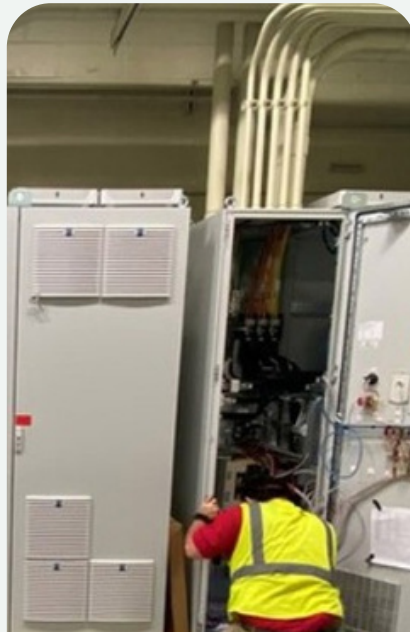
Installation & Commissioning of ABB VFDs – United Sugar Co., Jeddah
