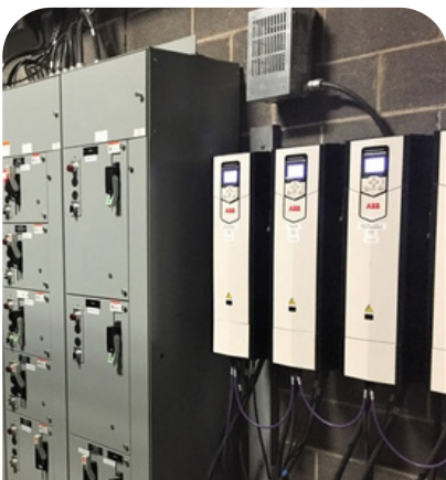
Installation & Commissioning of ABB VFDs – Al Safwa Cement Co., Jeddah
