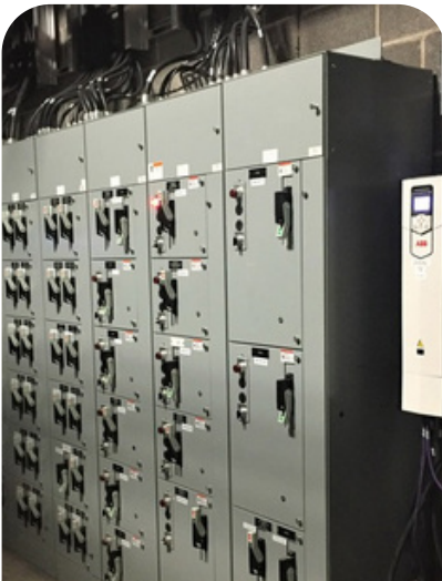
Installation & Commissioning of ABB VFDs – Aramco, Riyadh
